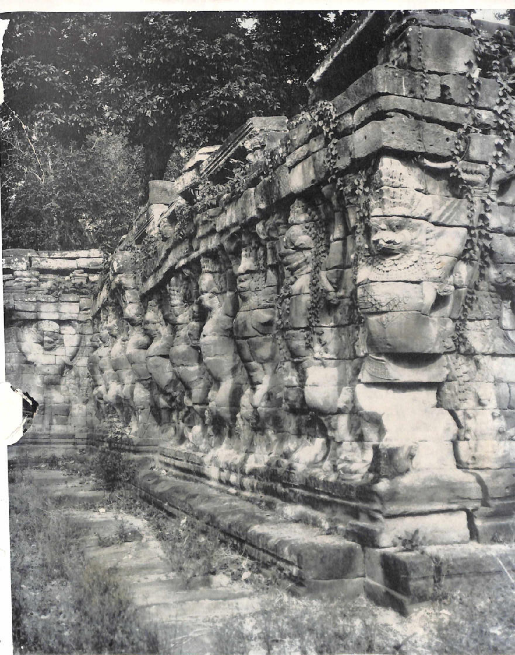
583. Garudas supporting the Royal Terrace
