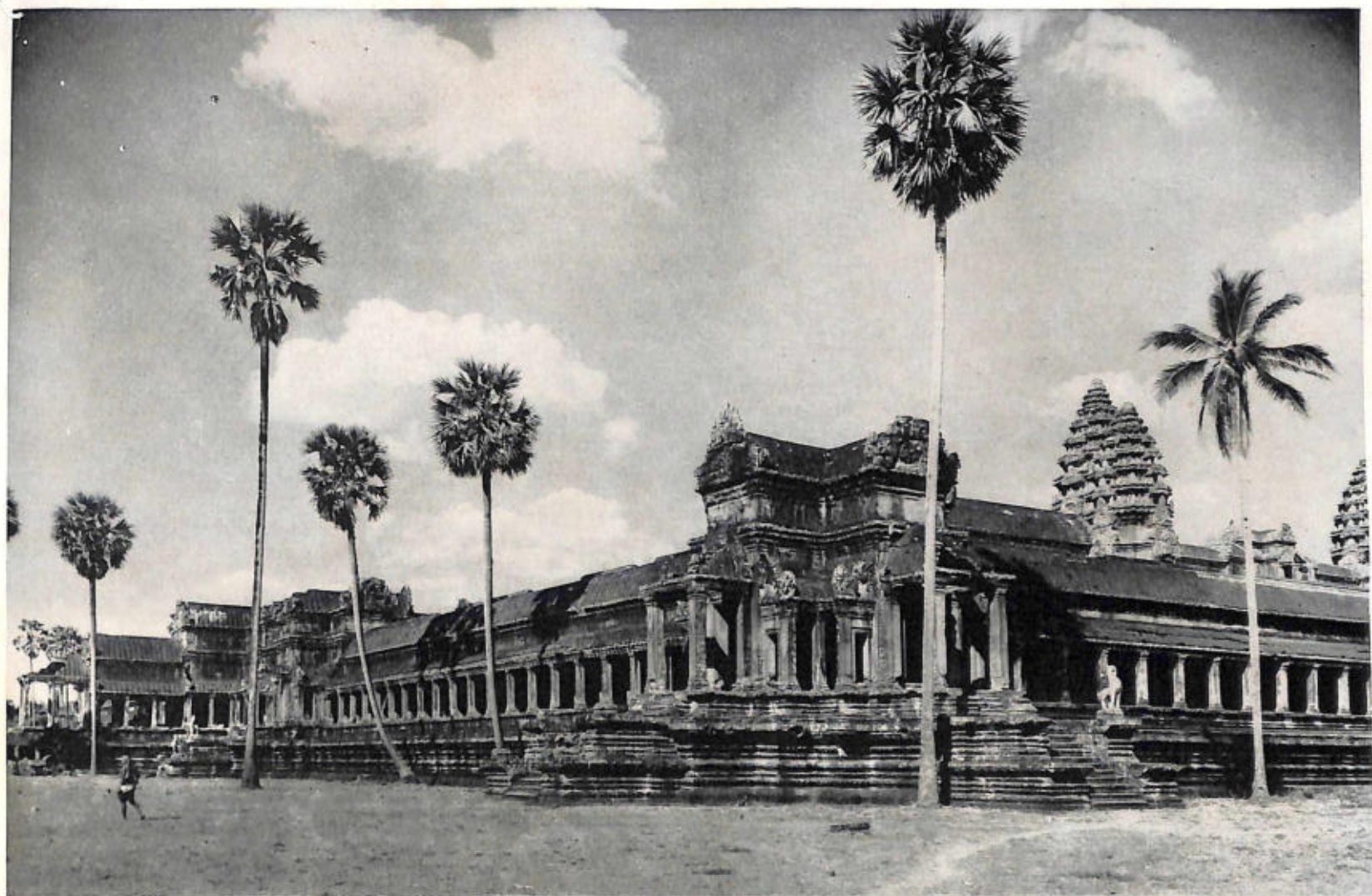
533a. Southwest corner
