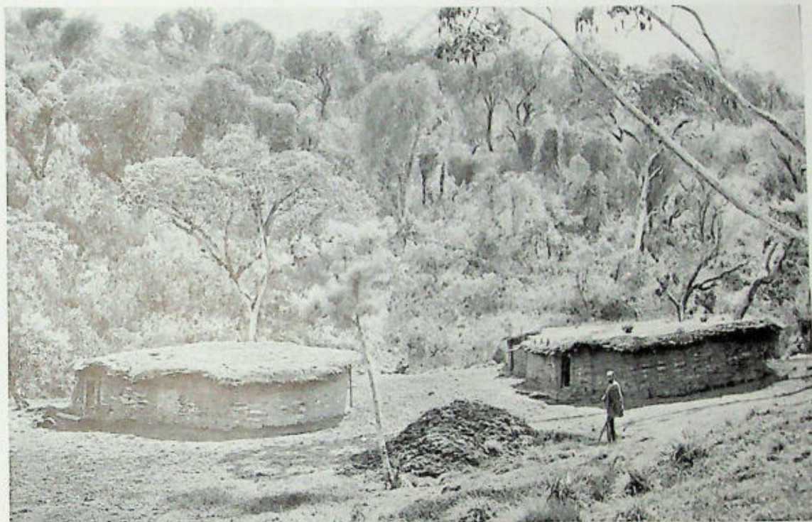
On the plateaus between the lands of the fiery sun and the temperate mountain zone the caravan came across these low huts, made on a framework of sticks, twigs and leaves and plastered with layers of cow dung which sheds the rain effectively. These huts are similar in structure to those of the Masai and many are also built in the caves on Mt. Elgon.
