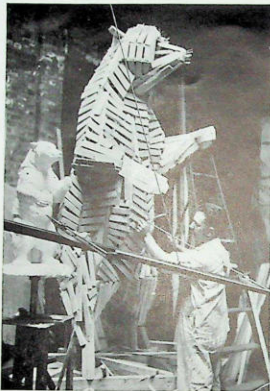
Building the structure of wood upon which the mold for the bronze will be made.
