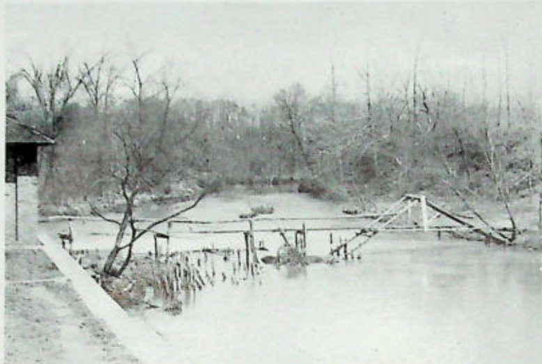
THE FOOT OF THE DAM
