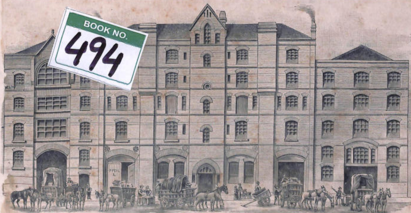
IRON AND TIMBER WAREHOUSES:—MACKLIN STREET, ST. GILES.
