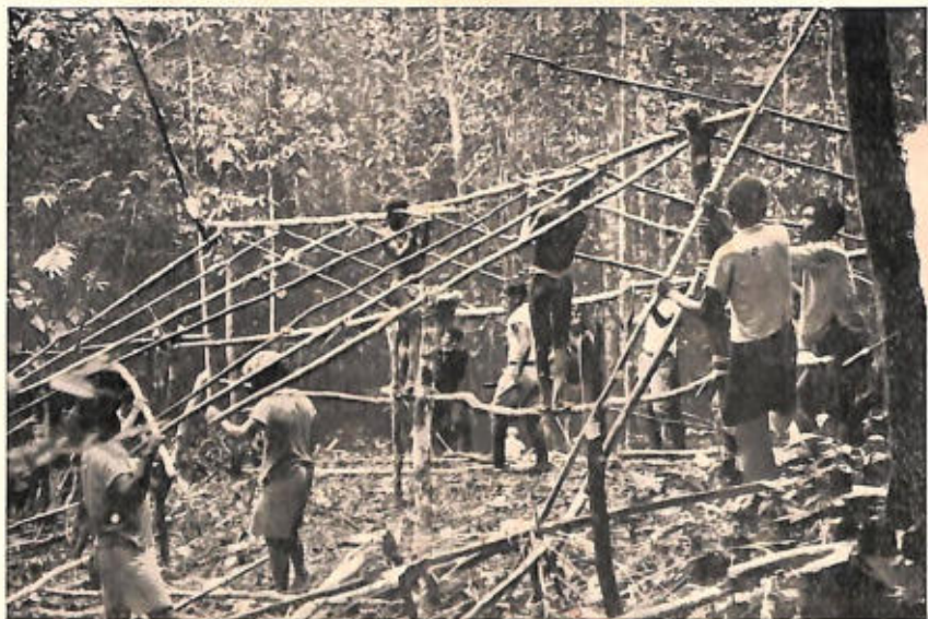
The poles go up for the framework of the tent.
