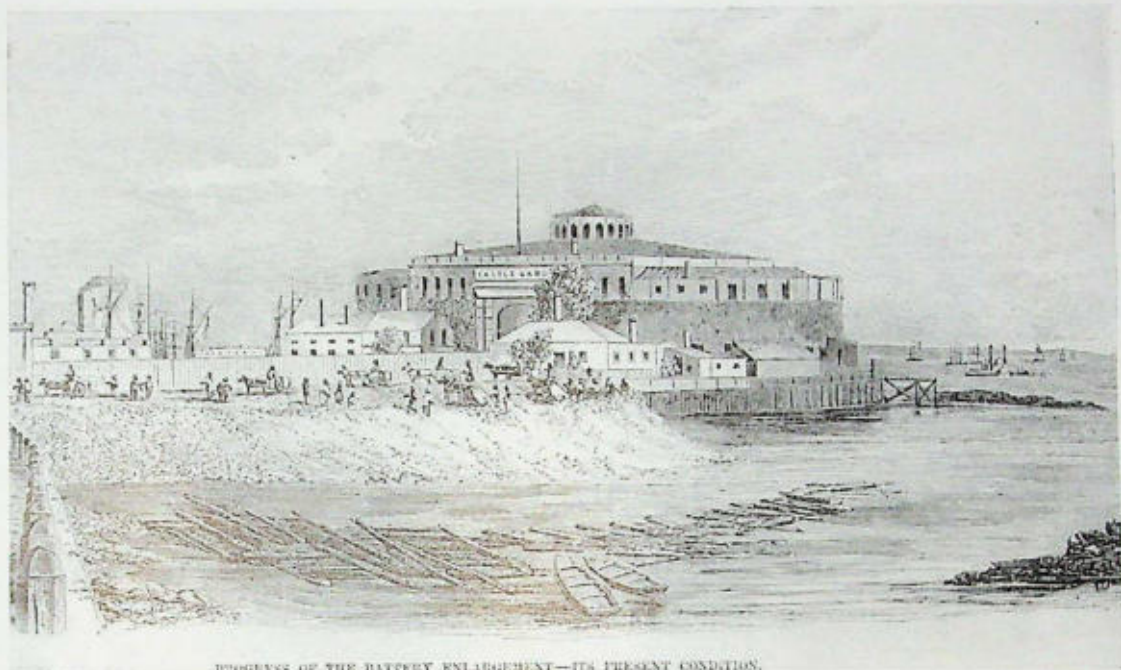
PROGRESS OF THE BATTERY ENLARGEMENT—ITS PRESENT CONDITION.
