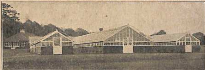
GROUP OF ORCHID HOUSES ERECTED FOR BARON BRUNO SCHRODER, AT THE DELL, ENGLEFIELD GREEN, SURREY, COMPLETE WITH DISPLAY CORRIDOR, POTTING HOUSES, STORES, BOILER HOUSE, OPEN SHEDS, WATER RESERVOIR, Etc. Etc
