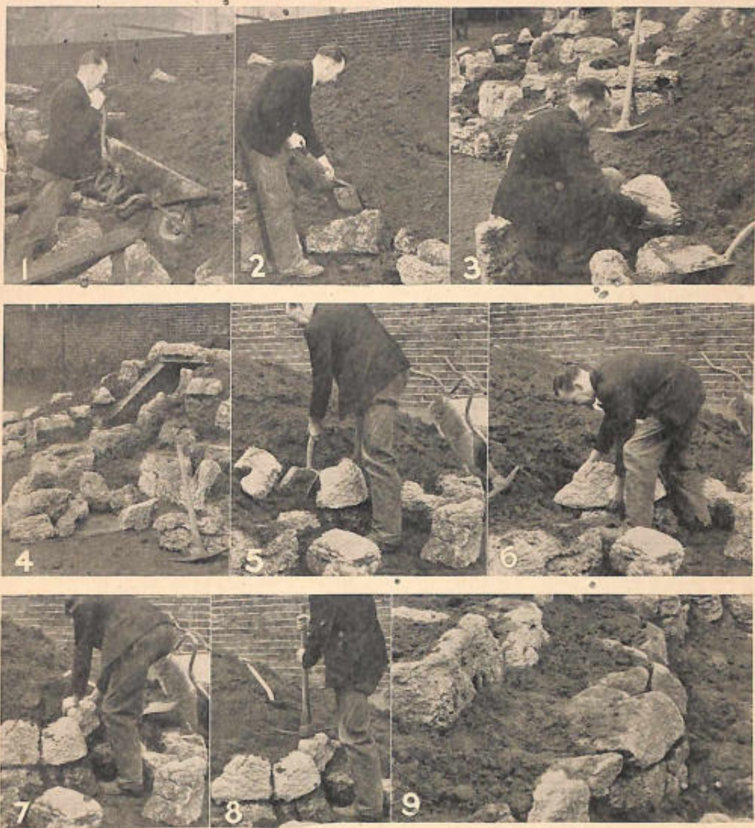
(1) Soil to build up the rockery can be wheeled on as work proceeds. (2) Make sure the soil is worked in well behind the stones. (3) The arrangement of the stones should be undertaken carefully. (4) Rocks should be placed on sacks when building takes place on a lawn. This will protect the grass. Note that an old air-raid shelter is being concealed by building this rock garden over it. (5) Soil being placed on a piece of rock to form a 'seating' for another piece. (6) The next rock being put in place. (7) Further rocks being added. (8) Firming of the rocks is important. (9) The rocks should be arranged in terraces.
