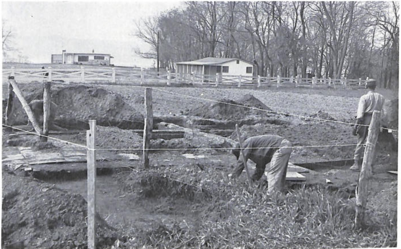
Figure 47.—FOUNDATION of Structure E (kitchen).
