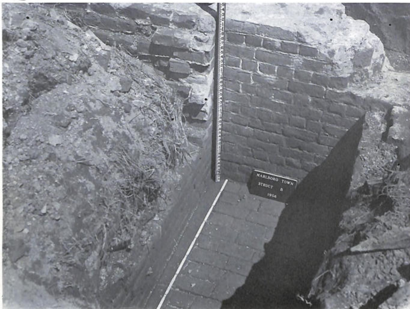
Figure 37.—CELLAR OF STRUCTURE B, showing remains of original cross wall at left and added cross wall at right. Mercer probably referred to the latter in 1749 in his account with Thomas Barry: "Underpinning and altering the cellar."
