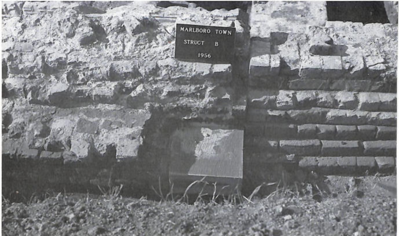
Figure 34.—SOUTHWEST CORNER OF STRUCTURE B. Piazza foundation extends to left, with red sandstone block at junction of piazza with main foundation. To the left of top of sign, molded red-sandstone trim can be seen which apparently surrounded the piazza. Bricks in front of trim appear to have been added later as step foundation. Brick buttressing of main-foundation footing appears at right.
