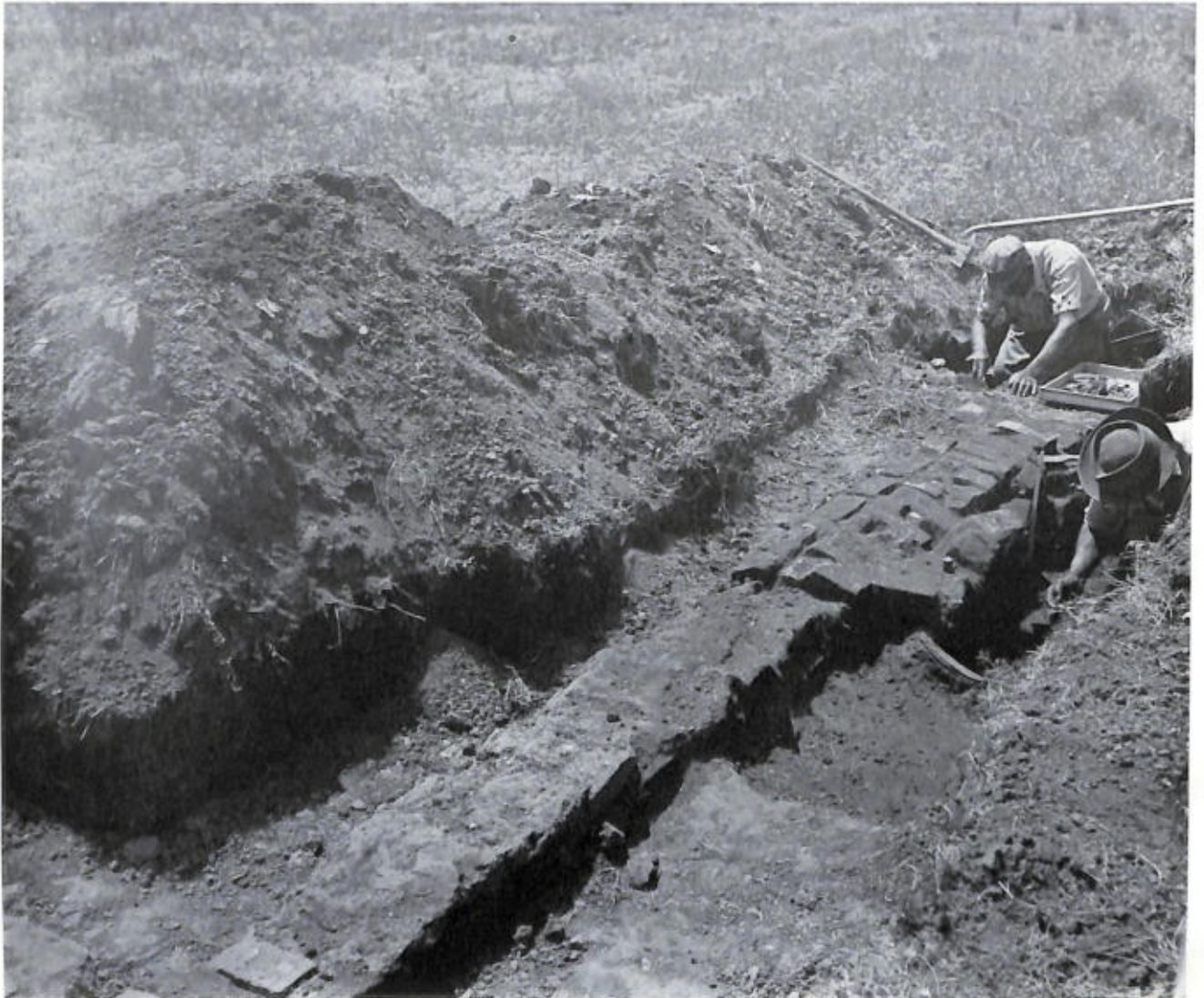
Figure 28.—WALL E, south of kitchen, showing gateway foundation.
