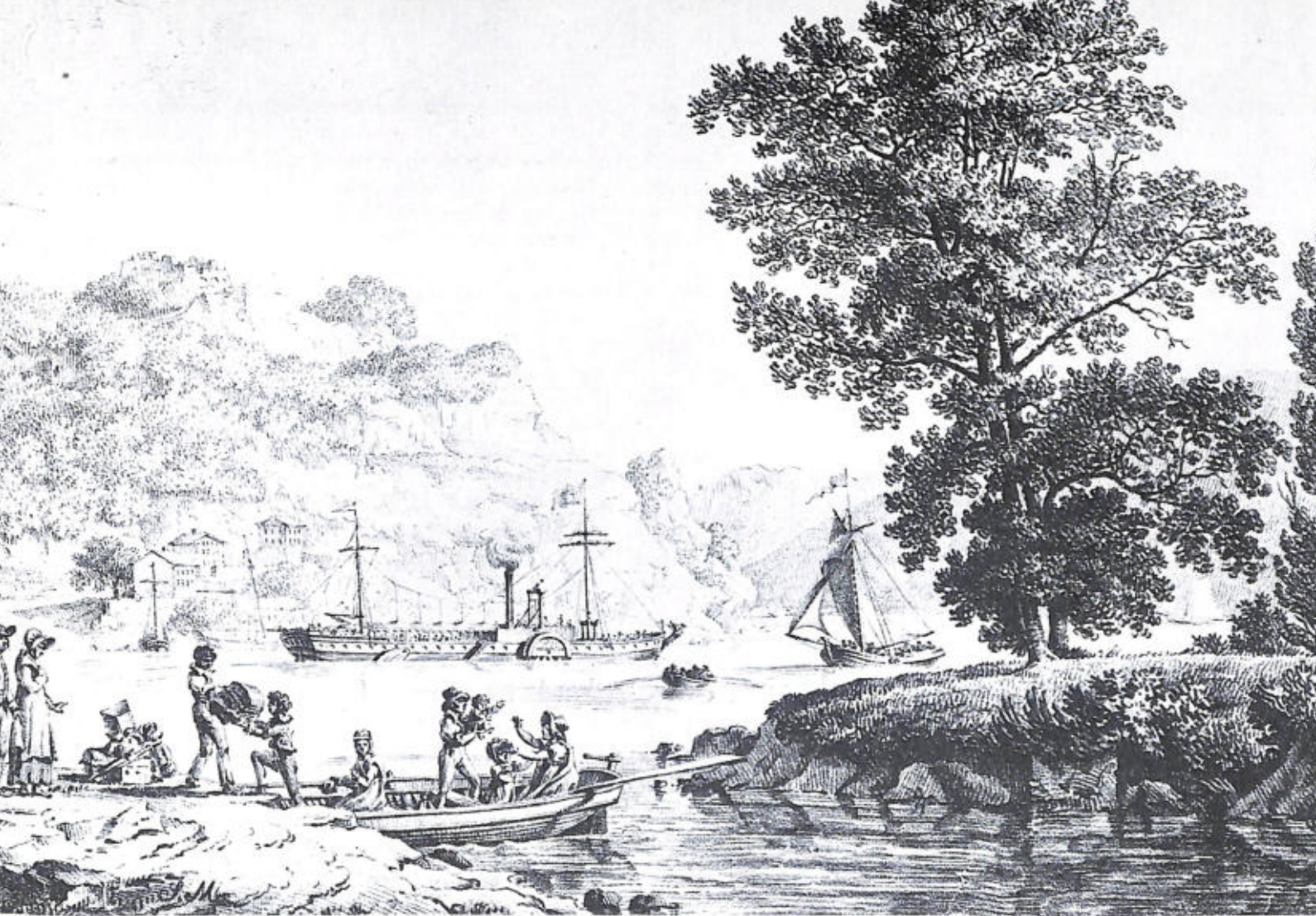
CONTEMPORARY VIEW OF FULTON'S STEAMBOAT. The North River (popularly known as the Clermont ) passing West Point, showing the vessel as rebuilt in 1807-08 with figurehead, wheelboxes, and leeboards. From a lithograph by F. Berthaux, Dijon, of a work attributed to Saint-Memin. (Photo courtesy of New York Public Library.)
