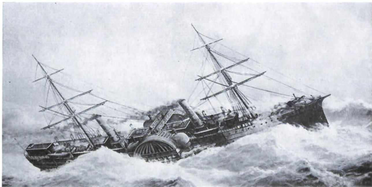
SIDE-PADDLE-WHEEL STEAMER Fulton , from a French print in the Watercraft Collection (USNM 160010). Built by Smith and Dimon in 1836 for the New York-Le Havre service, her register dimensions were 290' x 42'4" x 31'6", 2,300 tons. She was broken up in 1861. (Smithsonian photo 44638-c.)
