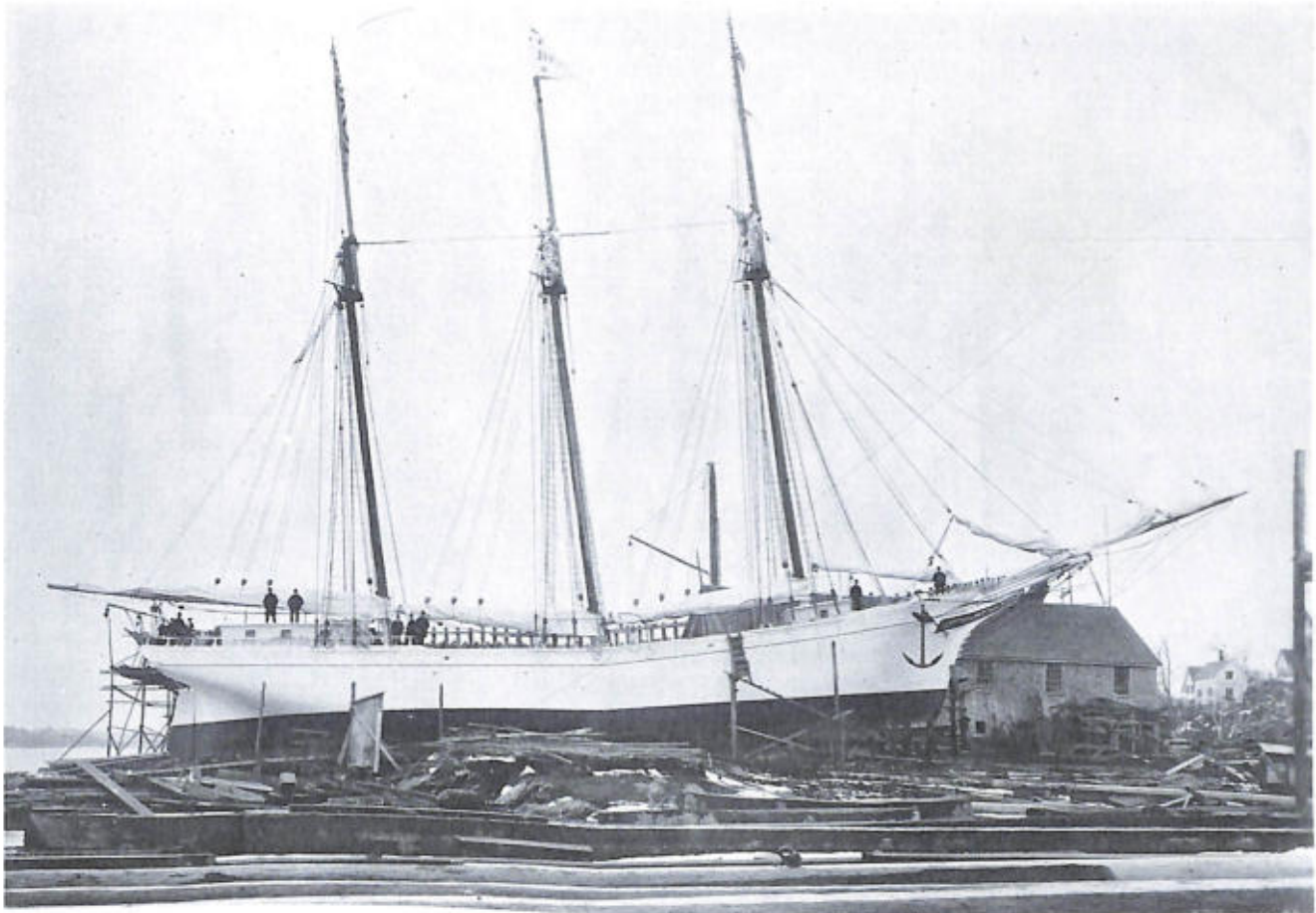
THE 3-MASTED SCHOONER Bertha Louise , of Fall River, Massachusetts, built by Kelly and Spear of Bath, Maine, and launched March 1, 1890. A typical New England 3-masted coasting schooner of the date, her register dimensions were 115.2' x 28.3' x 8.7', 231.42 gross tons. (Smithsonian photo 44872.)
