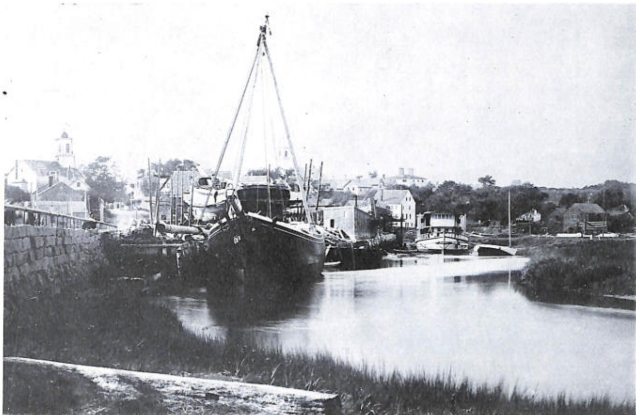
TARR AND JAMES SHIPYARD AT ESSEX, MASSACHUSETTS, ABOUT 1885, with one vessel in the water and another behind it on the ways. A new river steamer is in the background and other yards are beyond, with three ships on the ways. Center of village is to left, in background. Sheers and hoisting tackle are rigged to step the mainmast of the schooner in the foreground. The mast is alongside on the wharf. ( Smithsonian photo 44793-h. )
