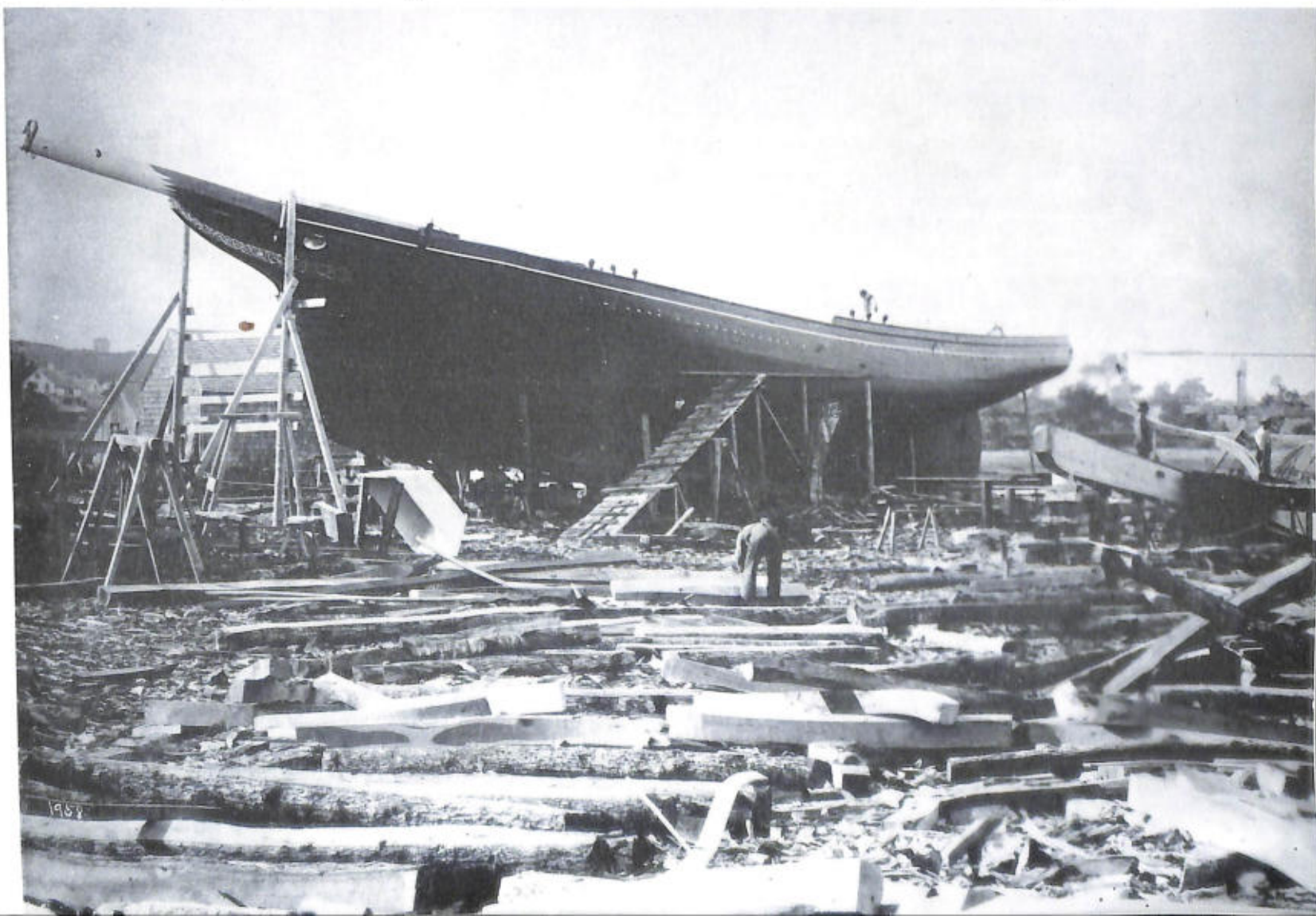
SCHOONER UNDER CONSTRUCTION AT ESSEX, MASSACHUSETTS, IN WILLARD A. BURNHAM'S YARD, 1882, the Belle Franklin . Her register dimensions were 78.6' x 22.2' x 8.1', 76 net tons. An excellent example of the "clipper" type, she was owned by John F. Wonson and Co., of Gloucester, Massachusetts. (Smithsonian photo 34911-c.)
