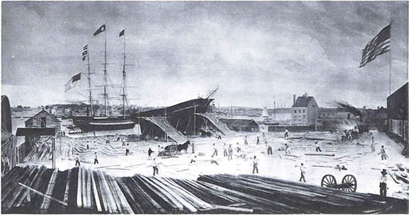
SMITH & DIMON SHIPYARD, NEW YORK, ABOUT 1831, FROM A CONTEMPORARY PAINTING. This firm was then a leading builder of packet ships, and later built Rainbow , Sea Witch and other famous clipper ships. A treadmill can be seen at the extreme left and a steam box at the extreme right. (Smithsonian photo 32914-c.)
