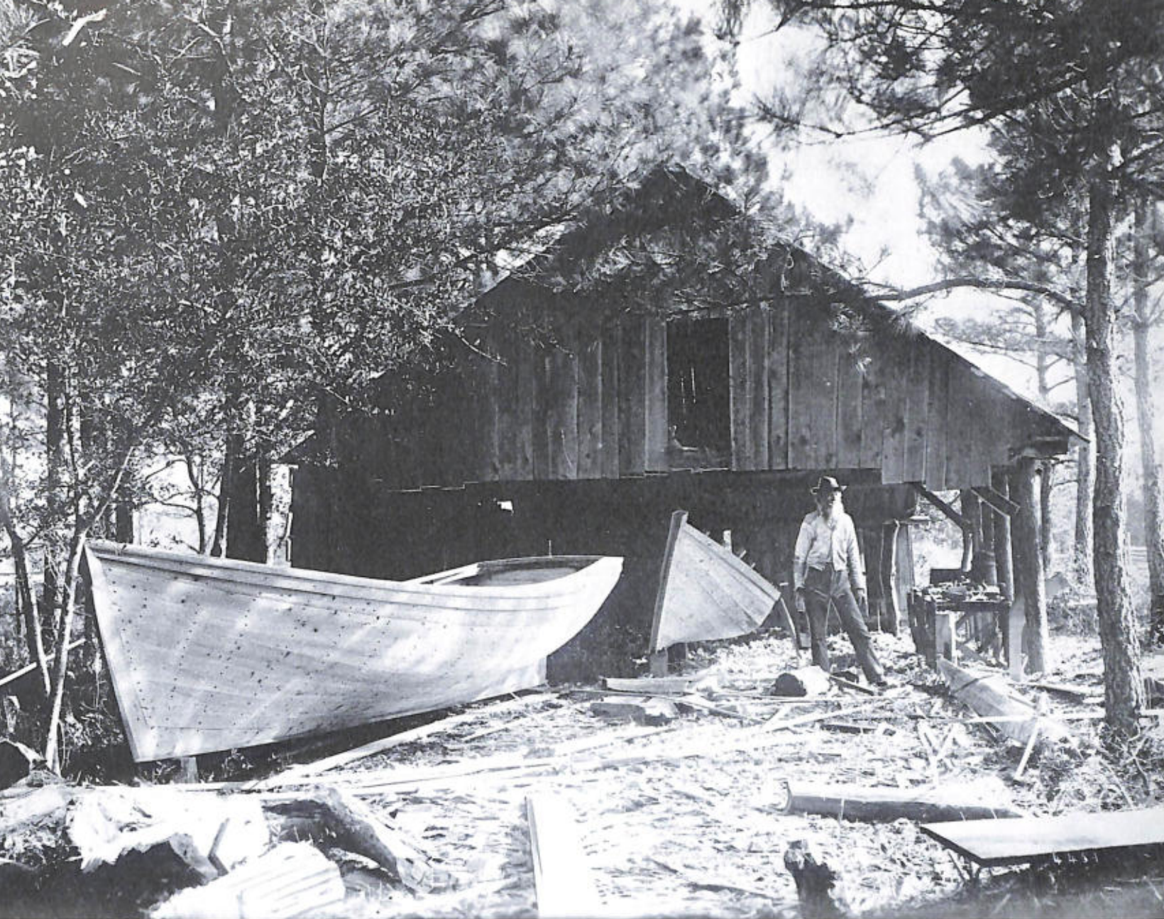
ALBERMARLE SOUND SHAD BOATS BEING BUILT AT ROANOKE ISLAND, NORTH CAROLINA, at the yard of the noted local builder, Washington Creef, in the 1890's. These boats, fitted with planked stern deadwoods, are large for their class. A good example of the simple boat shops in which these small fishing boats were built. ( Smithsonian photo 44793-f )
