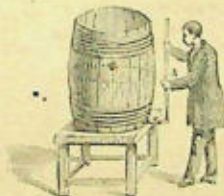
Fig. 122. — The water stops at A, at just the same level as in the cask.
