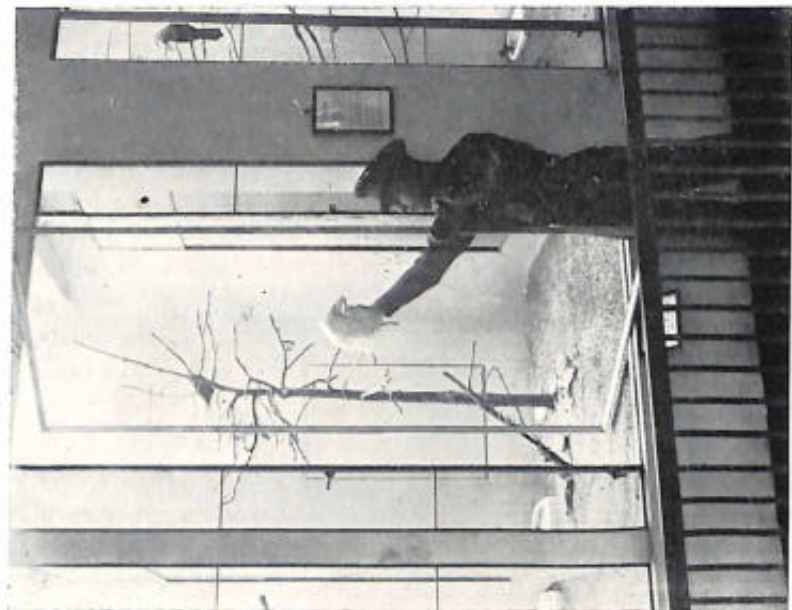
DETAIL OF THE PIVOTED GLASS CAGE FRONT. THE GLASS IS OPENED TO SHOW METHOD OF OPERATION. NOTE THE WIRE GRILLS ON EACH SIDE OF THE GLASS. THE METHOD OF LABELING IS ALSO SHOWN.
