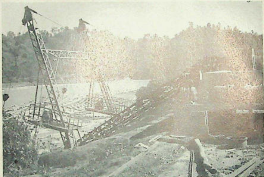
1. At the recently completed Karnaphuli Paper Mill, East Pakistan, bamboo will be used to produce 100 tons of pulp per day. Equipment shown was specially designed to lift rafted bundles of bamboo from the river to the flume, by way of which they will reach the mill.
