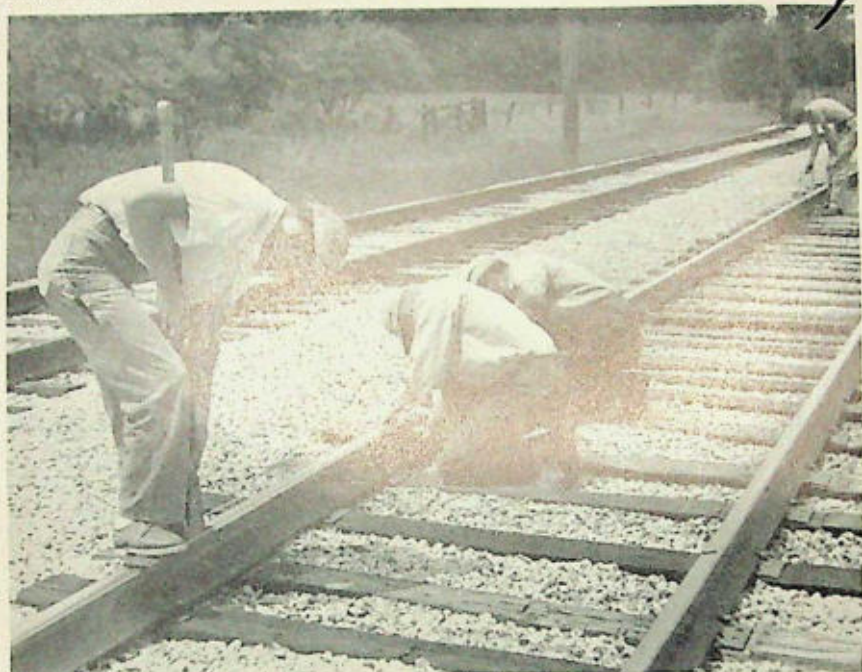
1. Baseline measurement for the triangulation network.
