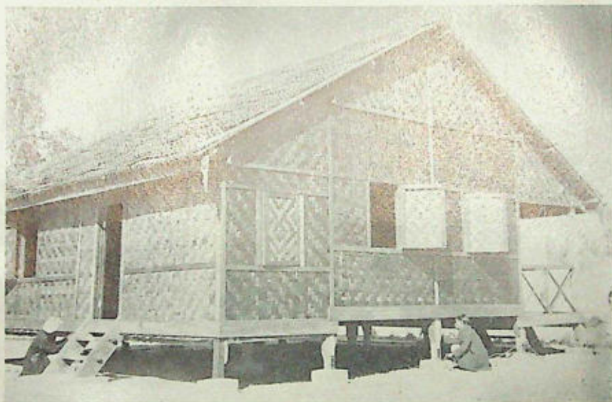
1. Hardwood-framed house with walls of bamboo matting and roof of bamboo shingles ( Bambusa polymorpha ). A modern adaptation developed in Burma.
