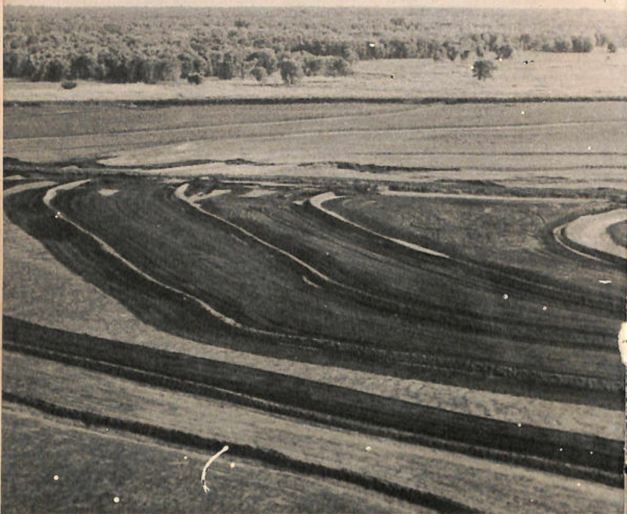
Land under development for the rice-growing project at Humpty Doo
