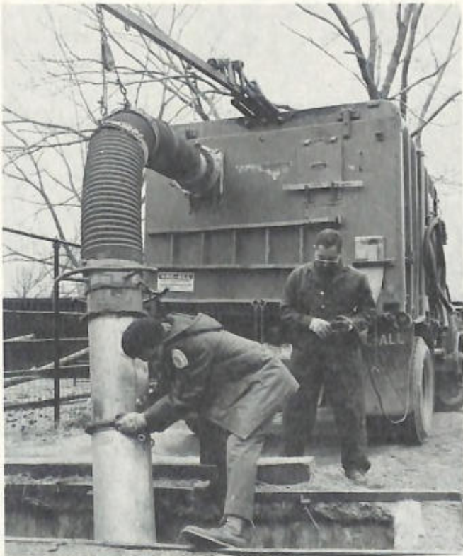
4. A large vacuum pipe is lowered into a trough in the kudu yards to remove excess water. This is one of many activities performed for the constant maintenance of the Zoo's animal exhibits.
