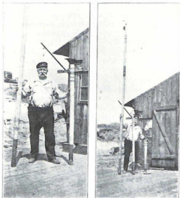
Figure 3.—ROD FLOATS SIMILAR to those used by Price at Clayton, Iowa, in 1881. (From Frederick Yancy Parker, "Mississippi River Gaging by Rod Floats," Professional Memoirs, Corps of Engineers, United States Army —1913, vol. 5.)
