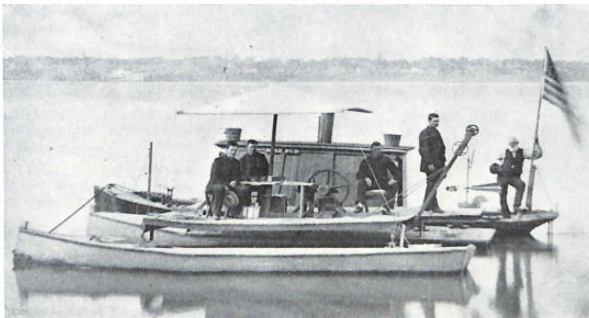
Figure 9.—PRICE'S STREAM-GAGING PLANT at Paducah, Kentucky, in 1882. Crew, from left to right: Dorst, Hoyt, McDonald, Price, and Hill. Note meter between Price and Hill. (Photo from scrapbook of W. G. Price.)
