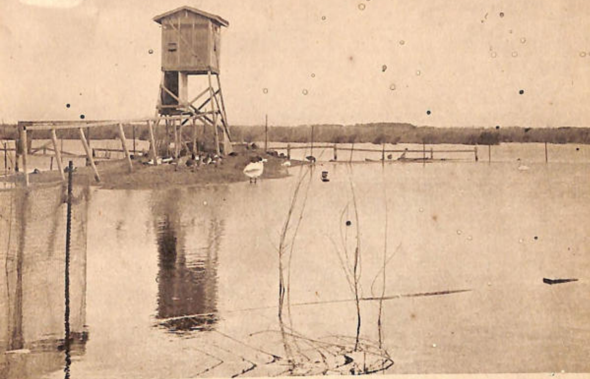
(Above) The observation tower at Delta. The effects of the rising level of Lake Manitoba •(see pages 74-79) are very evident.
